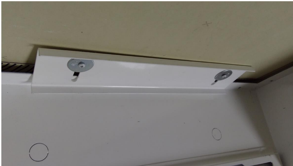
Figure 22: Mounting the Hard Ceiling Mounting Box
