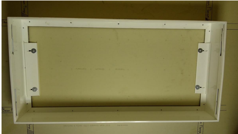
Figure 23: Temporarily Mounting of the Hard Ceiling Mounting Box
