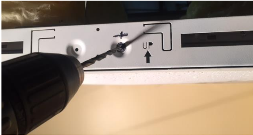
Figure 6: Drilling the Mounting Bracket
