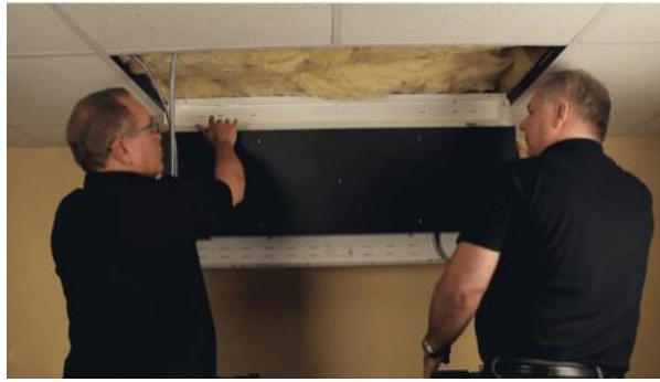
Figure 11: Preparing to Connect Power
