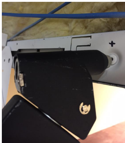
Figure 7: Riveting the Mounting Bracket
