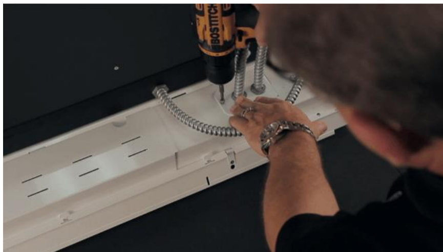
Figure 16: Completing the Wiring
