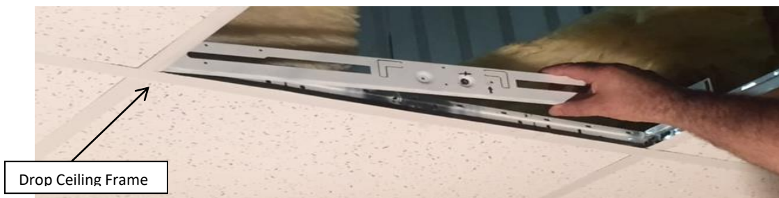
Figure 5: Mounting Bracket Installation
