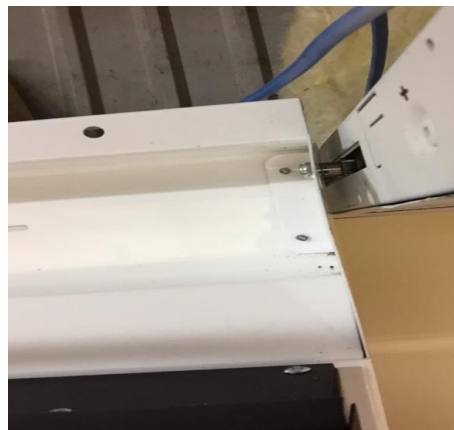
Figure 10: Fixture Hanging from Ceiling
