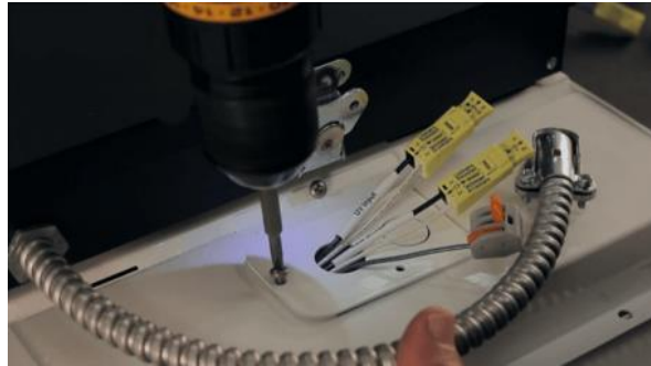
Figure 12: Removing the Electrical Access Plate
