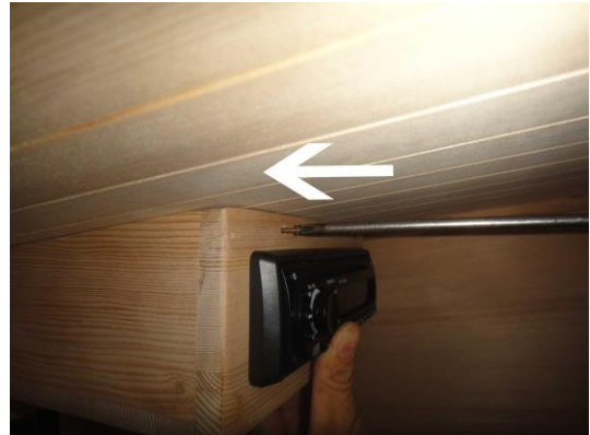
FIG 15.4 Screw wood housing to sauna room
