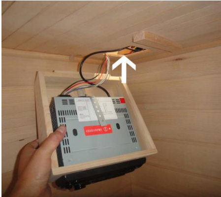
FIG 15.3 Feed the wires up through the roof
